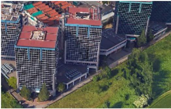
Figure 9: Tucide towers current status
