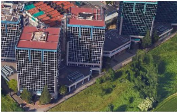
Figure 20: Tucidade towers before renovations
